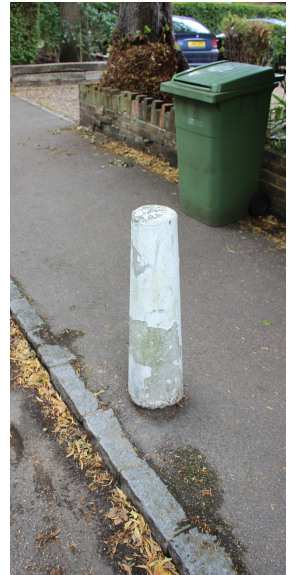
6f Concrete bollards
